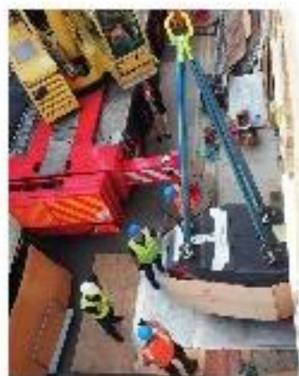
The scanner is craned into the clinic
