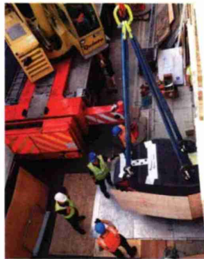
The scanner is craned into the clinic
